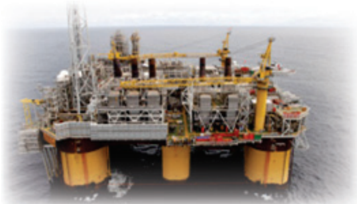
Planta Off-Shore (Noruega) Off-Shore plant (Norway)
